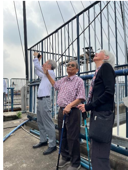
Mr. Ghoshal explaining the tower anchorage
