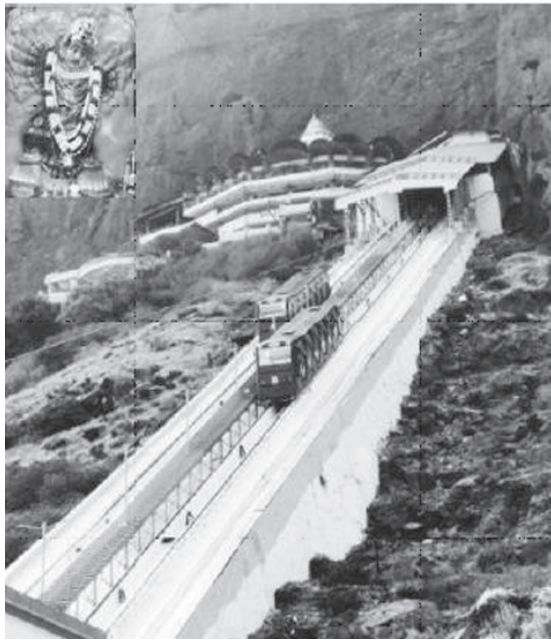
Saptashrungi Devi Temple Funicular Railway in Operation
