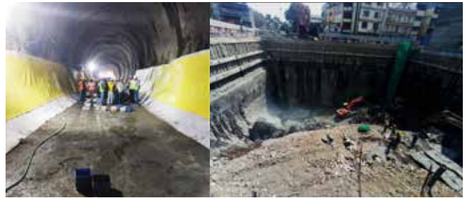
Figure 6: Tunnel inside view and a station top view of excavation
