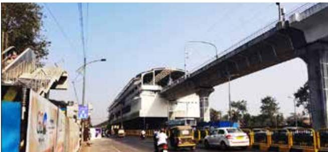
Figure 3: Typical elevated metro station and viaduct
