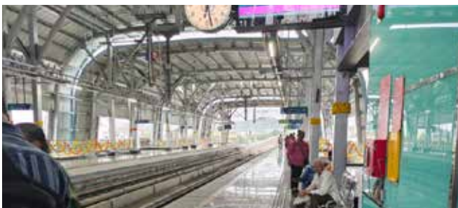
Figure 4: Typical inside view of a metro station
