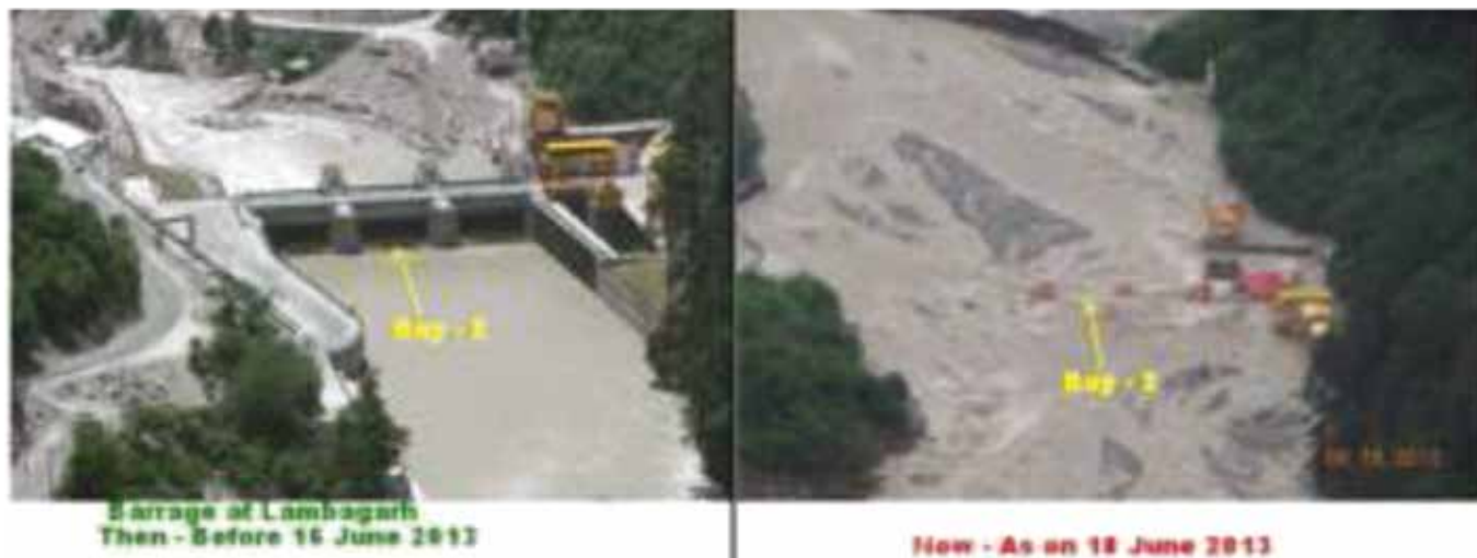
Figure-1 Aggradation Due to Landslides in 2013 Flood in Uttarakhand
