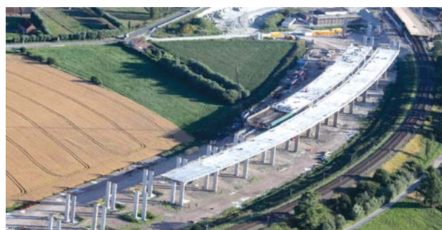
Fig.5. Construction of A11 highway bridge (Photo: Jan de Nul Group).
