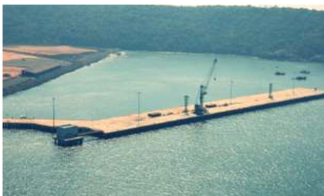
Bird's Eye View of Cargo Jetty with Container Yard in Background
