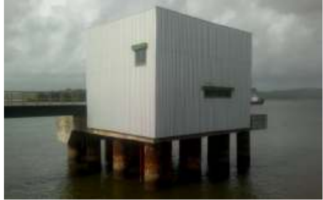
Fire Water Pump House on Mooring Dolphin
