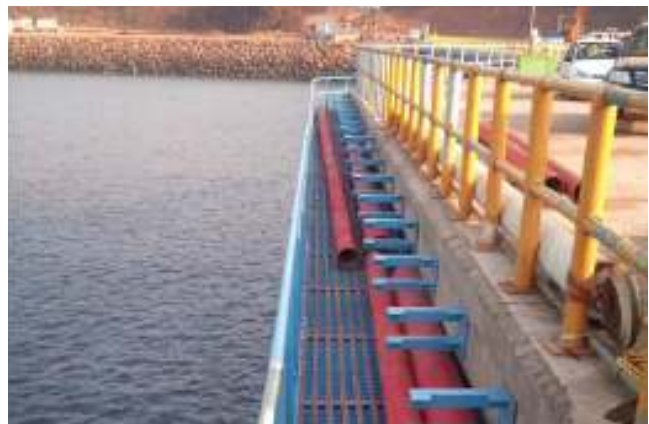
Utility Catwalk along the Approach Jetty
