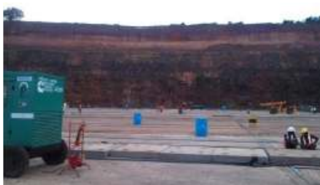
A View of Repair Yard Benching 60m High
