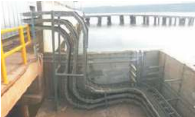
Transfer of Electrical Cables from Landside to Marine Side
