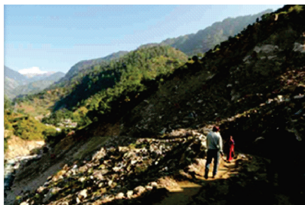
Landslides along the National Highway in Uttarkashi District due to the 2013 floods.
