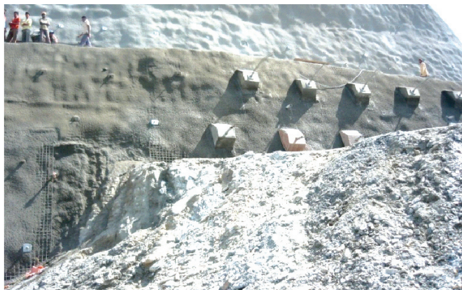
Slope stabilisation in powerhouse of Alakhnanda Hydro Power Plant
