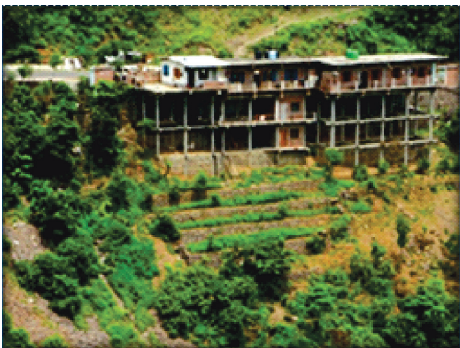
Building near Teen Dhar in District Tehri (Gharwal) near NH 58
