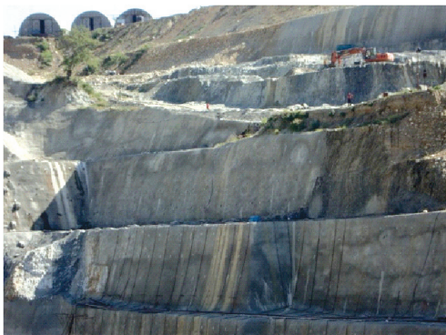
Slope stabilisation in power house of Alakhnanda Hydro Power Plant
