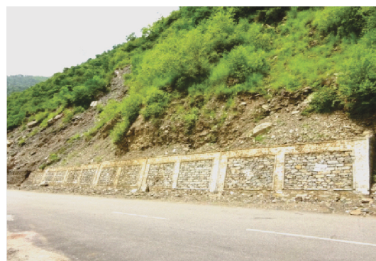
Toe wall along NH 58 near Rudraprayag
