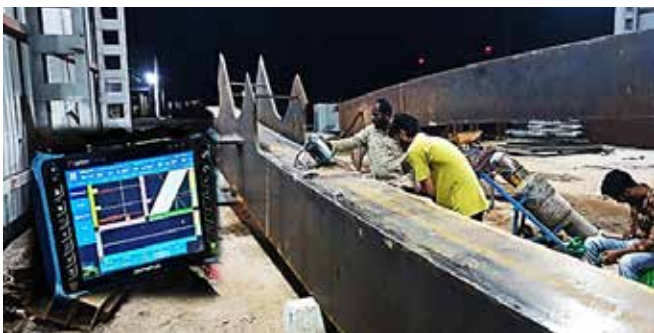
Fabrication of Lift Span and Tower – Weld Inspection by PAUT.
