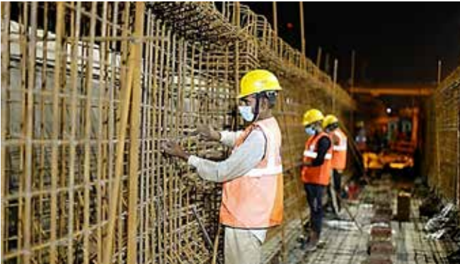
Namo Bharat casting yard
