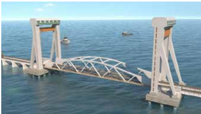
Reconstructed Pamban Bridge Including Navigational Lift Span
