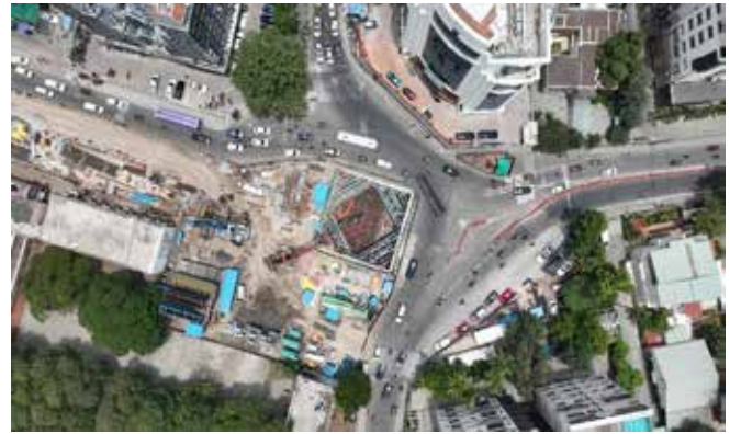
Traffic arrangement at Sterling Road junction
