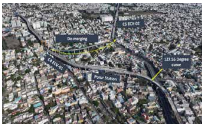
Intersection of Corridor 4&5
