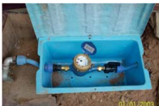
Installation of Consumer Meter
