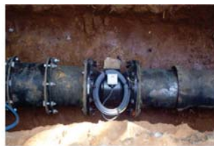
Installation of DMA Meter
