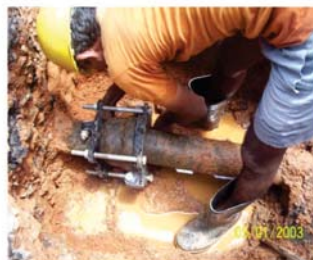
Leak Repair using Clamp
