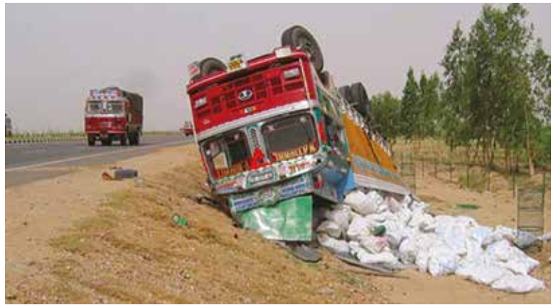
Un-protected side slopes, with no hard shoulder markings, that result in loaded trucks toppling over.
