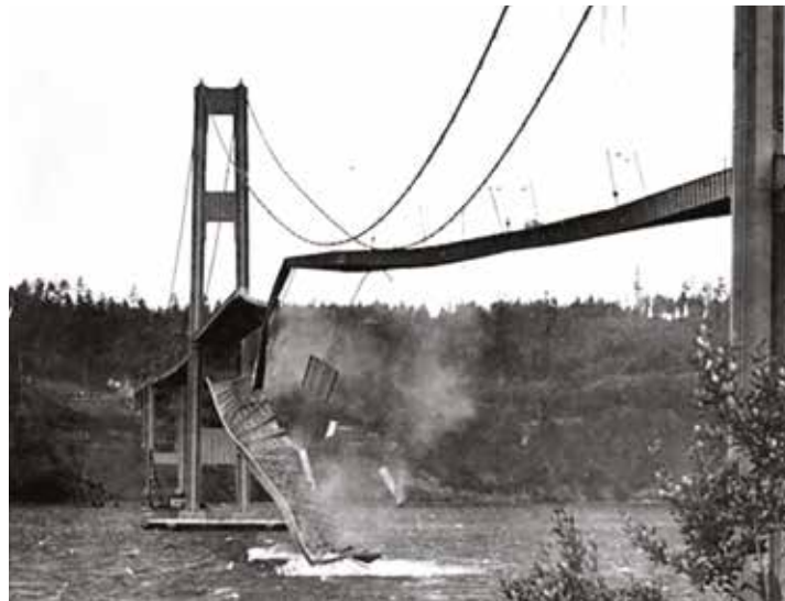
Collapse of Tacoma Narrows Bridge
