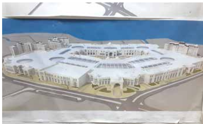
Photo-2: Vendome Mall Aerial View (courtesy- CRC)
