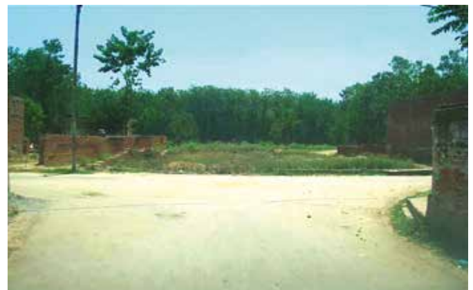
Poor visibility on both sides at a junction. Mirrors needs to be provided.
