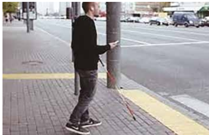
Figure 16: Intersection Design for Vision Impaired (notice the yellow mat for touch and feel)
