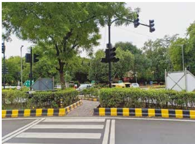
Figure 3: Signs are Non-Standard – Obstruct Sight Distance
