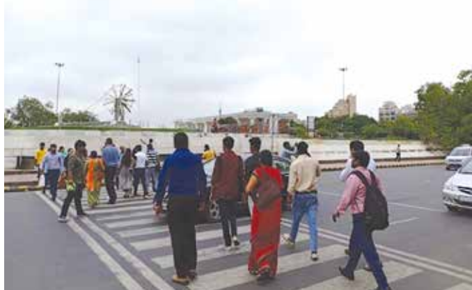
Figure 5: Lack of Stop Bar at Signalized Junctions (a car is in the path of pedestrians)
