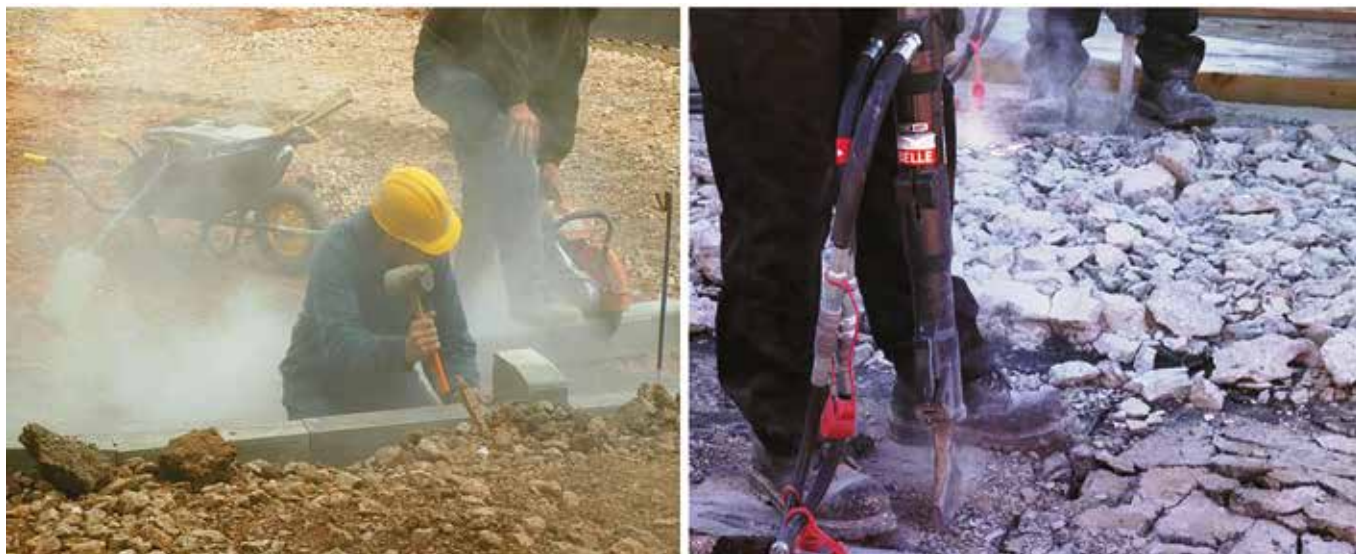
Figure 2: Typical Construction and Demolition activities, releasing concrete dust [5].
