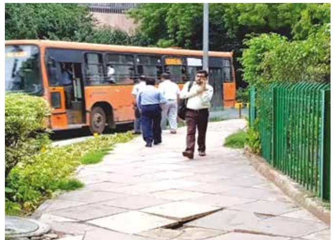
Figure 2: Fixing of Uneven Footpath
