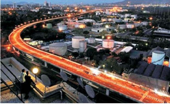
Mumbai's Eastern Freeway: Built to reduce travel time between South Mumbai and the Eastern suburbs, it connects P D'Mello Road to the Eastern Express Highway at Ghatkopar and covers a distance of 16.8km.
