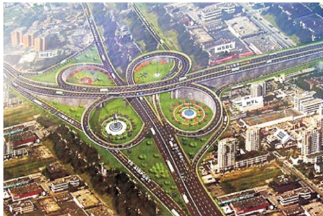
The Kathipura interchange is the largest cloverleaf flyover in Asia, situated at Alandur in Chennai.
