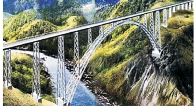
Chenab River Railway Bridge: Expected to complete by 2019, it will be the highest railway bridge in the world, over river Chenab, 359 meters above the river bed in Katra, Jammu-Kashmir. The 1.3km-long bridge is a part of the 73km-long Katra-Dharam section of the Udhampur-Srinagar-Baramulla Rail Link (USBRL) project.
