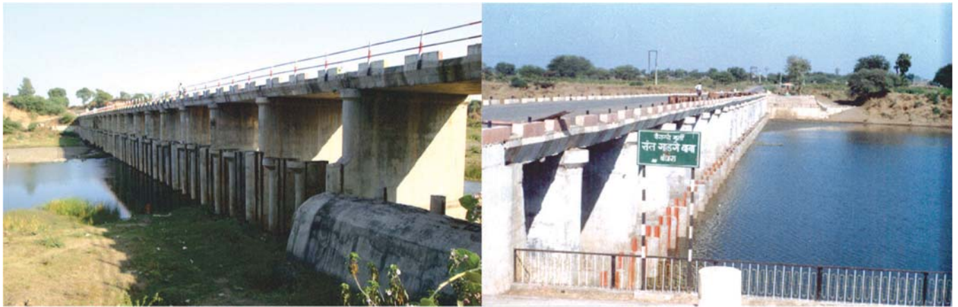
Bridge cum Bandhara
