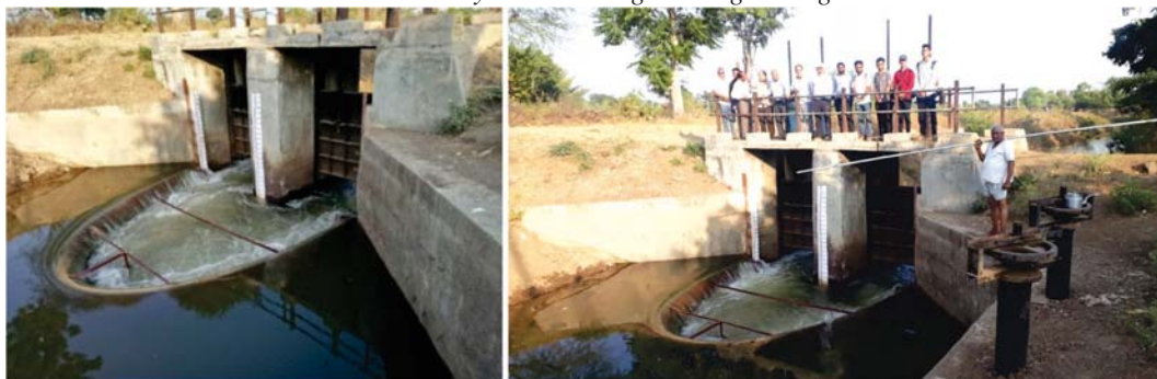
Study of flow over the elliptical weirs at Chandrabhaga Canal
