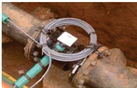
Installation of Flow Meter
