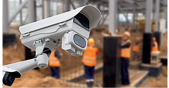
Photo-1: Construction site monitoring
