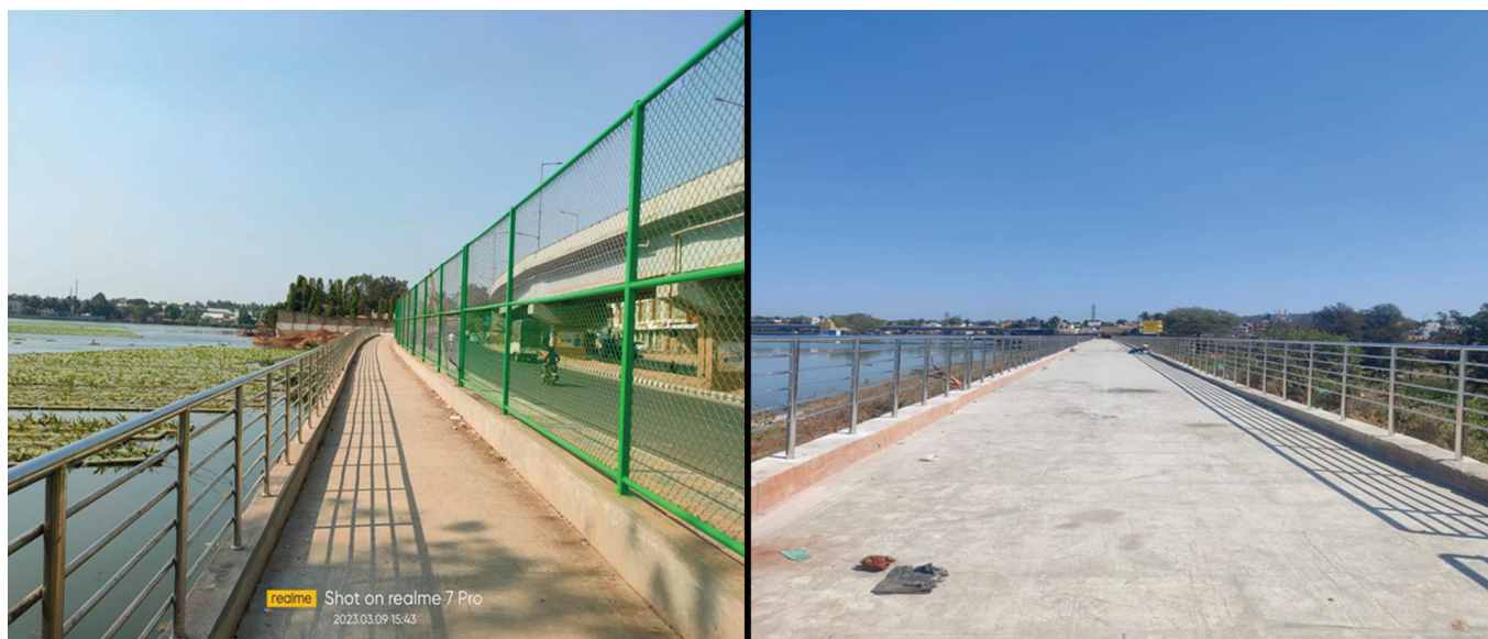
Photographs 5& 6: Lake Edge After Construction of Pathway Dam Wall after Beautification
