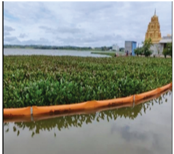
Photographs 3 & 4: JMS Trash barriers arresting floating matter from entering into the water body
