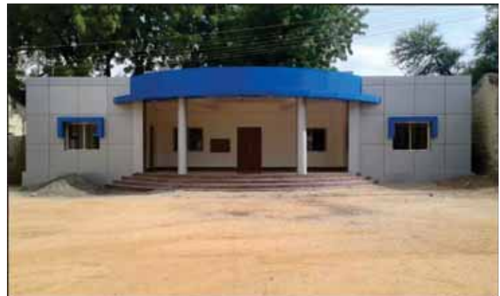
Figure 11 Master Control Station and Training Center
