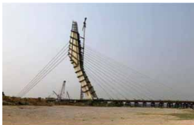
Figure 6: Wazirabad's Signature Bridge in Delhi
