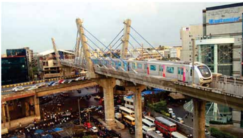
Figure 7. Views of monitored cable stayed bridge of Mumbai Metro over the Western Express Highway.
