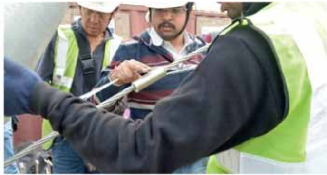
Figure 13. Sensors being placed on the cable strand before stressing
