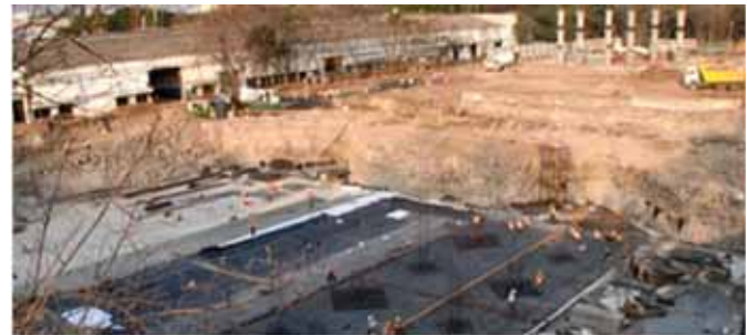
Figure 2: Remote Monitoring using PTZ Camera at Pune (2012)
