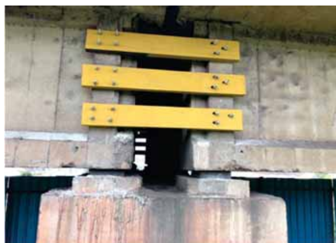
Fig 4:- Steel plate Ties between Two Girders.
