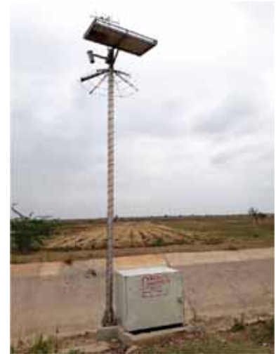
Figure 3 Typical Installation of Solar Powered Integrated Gate
