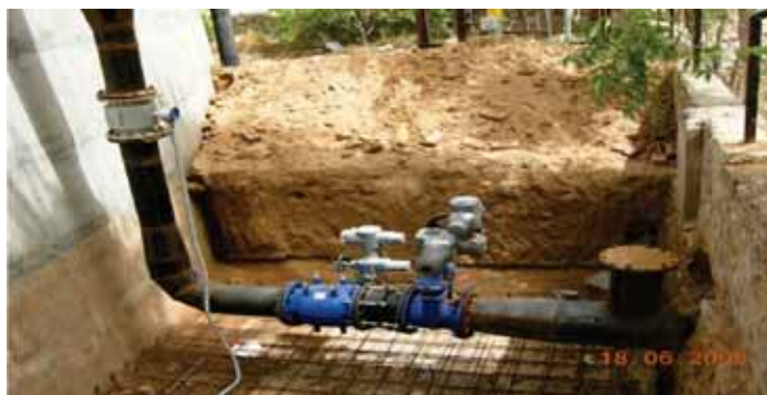
Flow Control Arrangement
