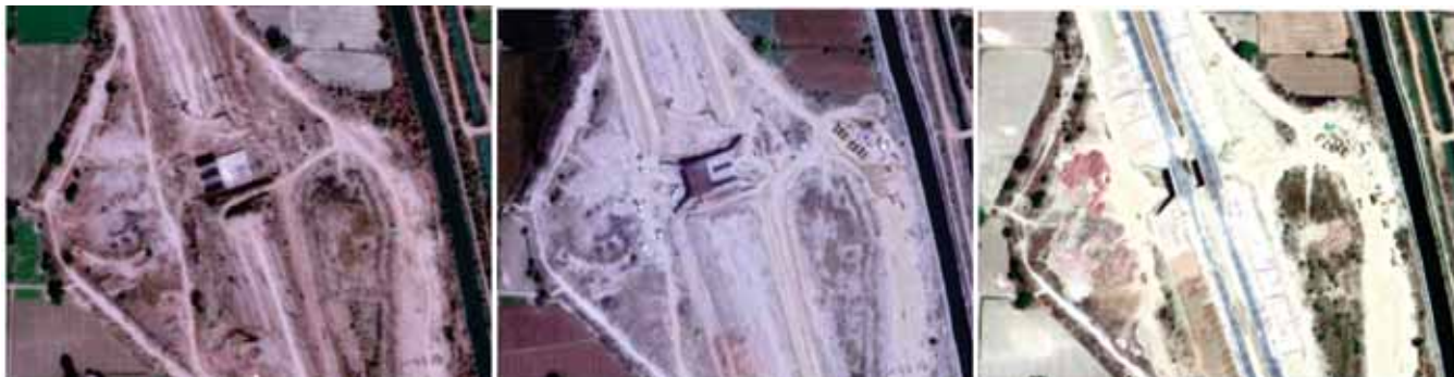
Stage 1 of Surface Preparation
