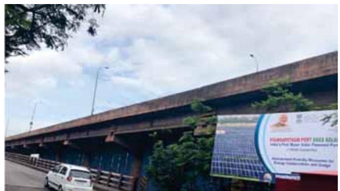
Figure-1: VISHAKHAPATNAM PORT TRUST BRIDGE
