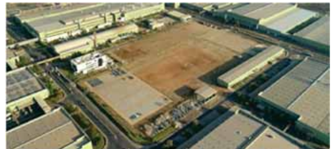
Figure 3: Site Planning using Drone Survey (2019)
