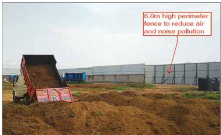
Exhibit 07: Site perimeter wind breaker
