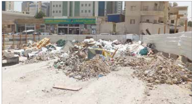
Photo 07: Waste Materials at a construction site.
