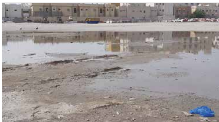
Photo 05: Stagnant wastewater at a sewer line extension work or well point dewatering system
