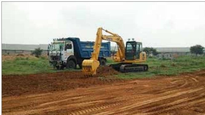
Exhibit 01: Removal of top soil
