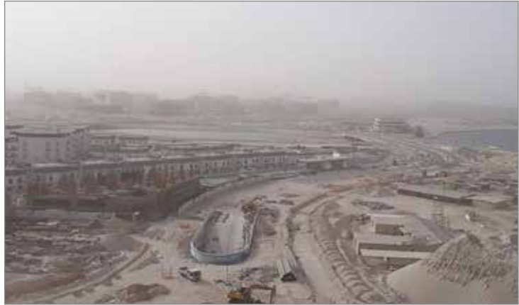
Photo 01: Dusty Environment in a construction area
