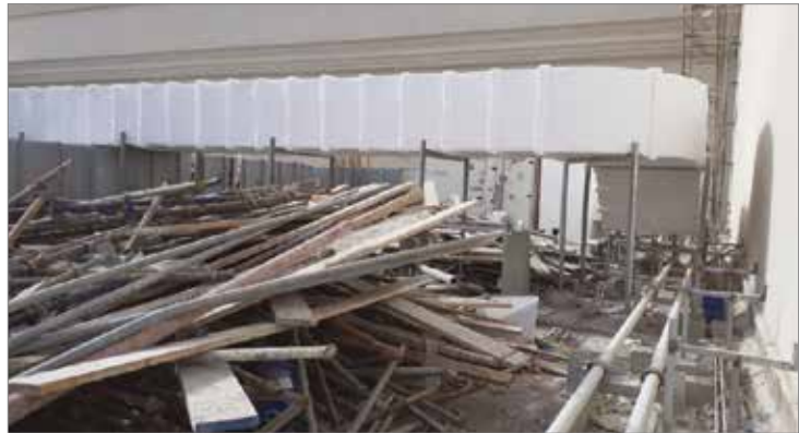
Photo 06: Waste Environment in a building construction site
