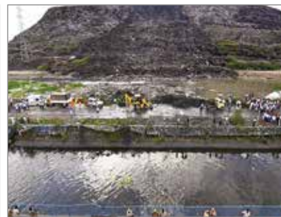
Drain flowing adjacent to Ghazipur dumpsite
