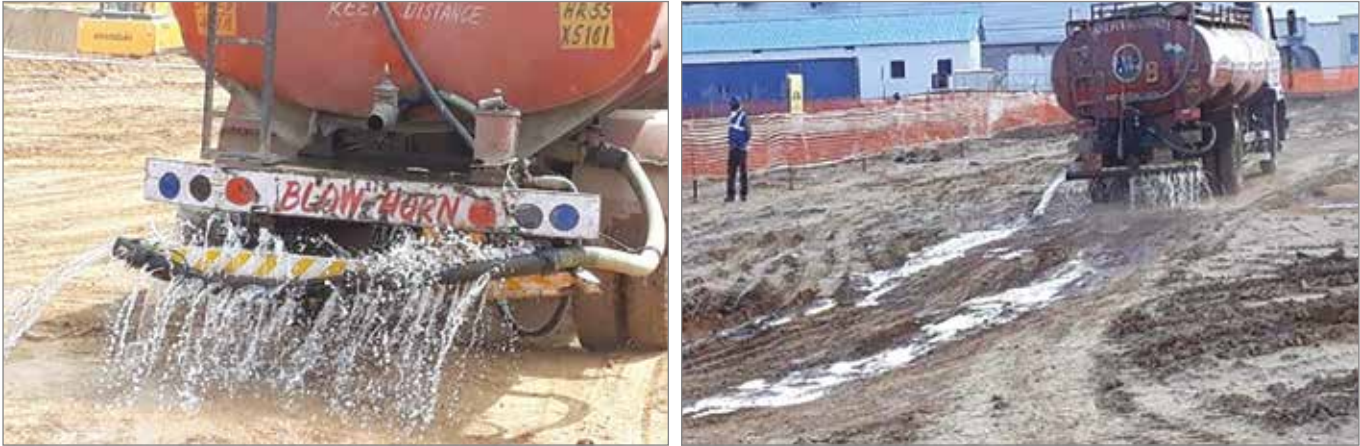
Exhibit 05: Water being sprinkled on an access road to suppress dust
