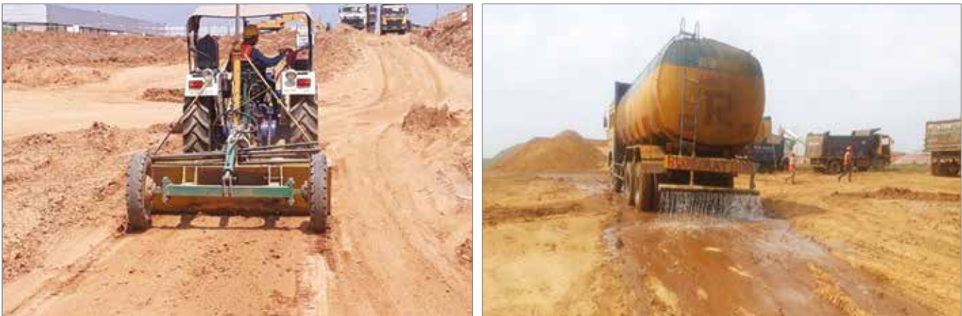
Exhibit 06: Water being sprinkled on an access road to suppress dust
