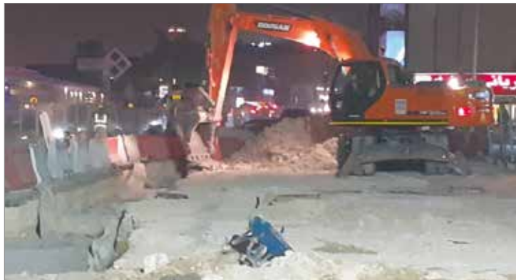
Photo 04: Pollution -Noise, Air & Dust, in a construction area
