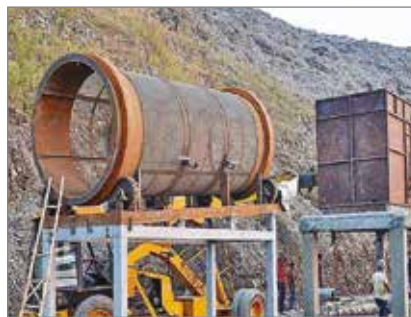
Tromel for Biomineral at Ghazipur dumpsite
