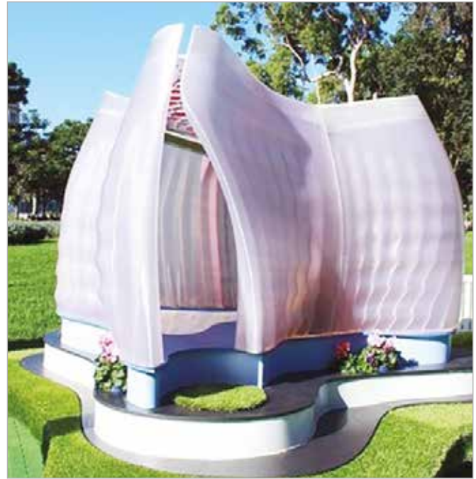
Kooky Cubby was designed by FMSA Architecture and manufactured with 3D printing technology developed by the Architectural Robotics Lab at RMIT University. While the details and specifications remain undisclosed, the structure can be bid on starting at $6,000.
