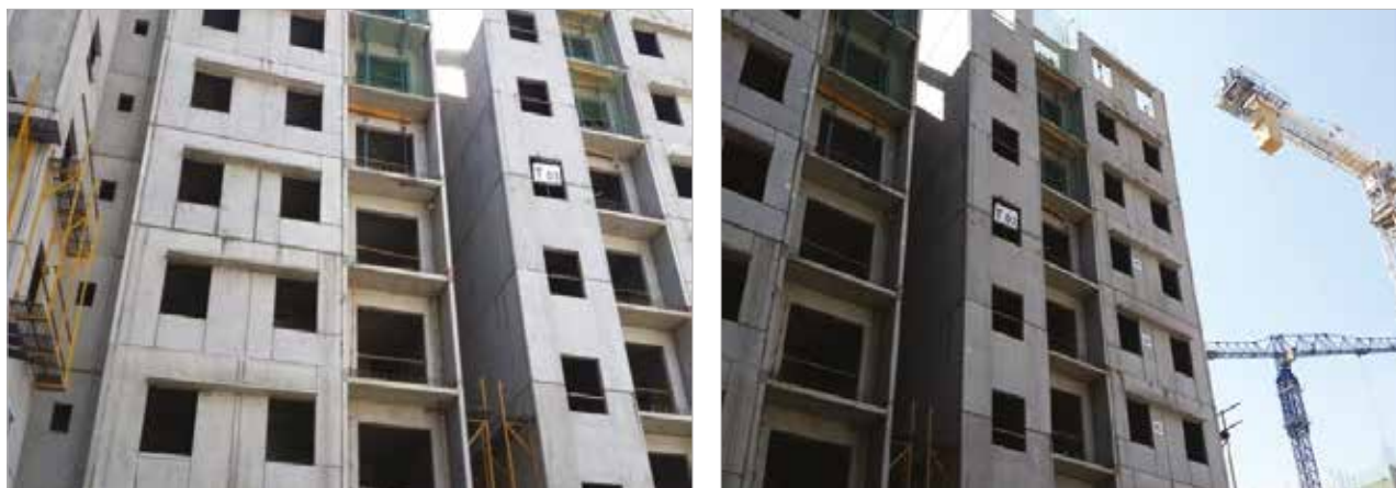
Precast construction - under erection at Peenya, Bengaluru – Tata Housing
