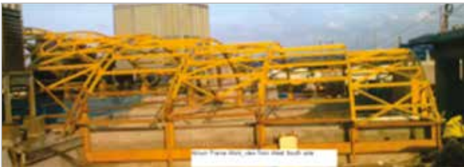
Atrium roof structure
