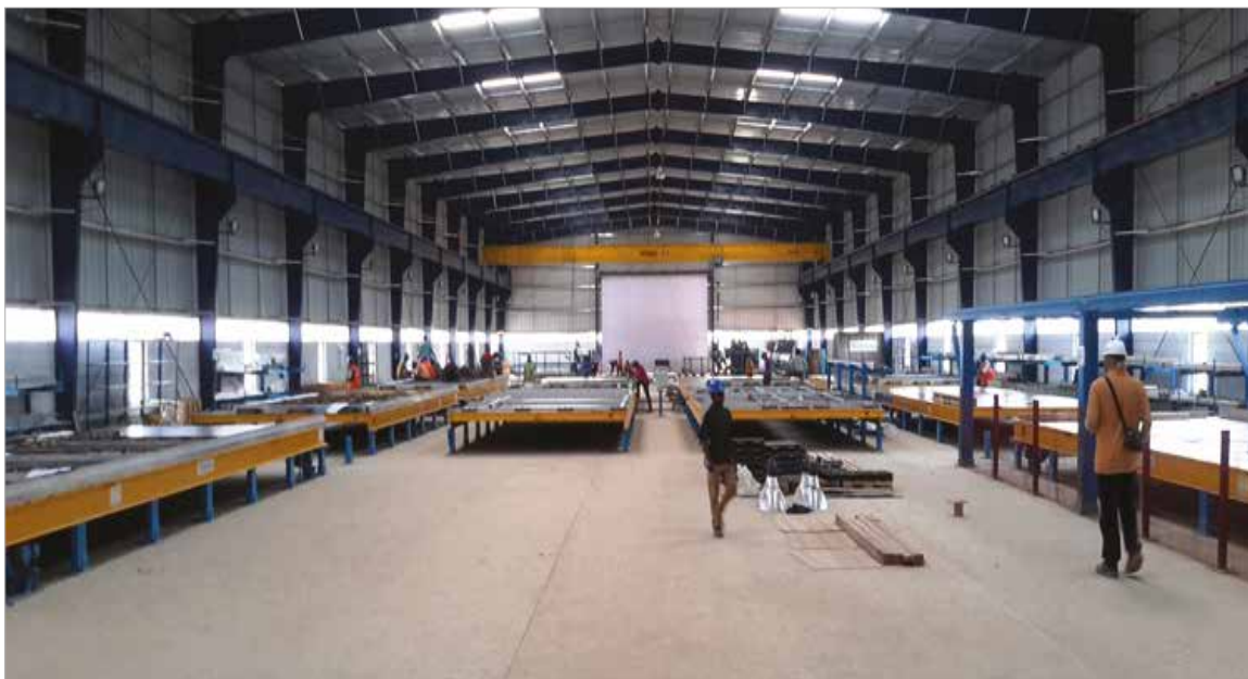
Carousel plant at New Haven, Peenya, Bengaluru, Tata Housing
