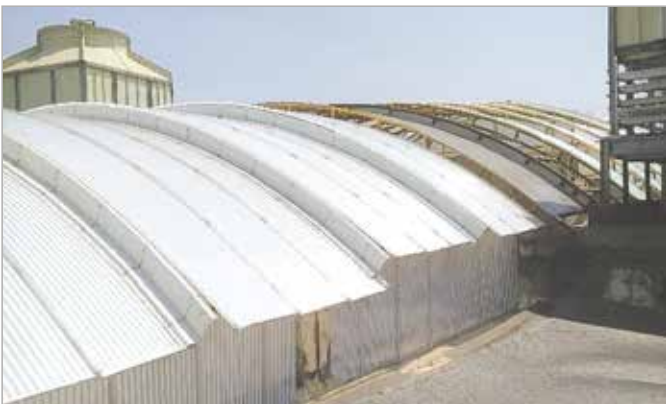
View of atrium roof
