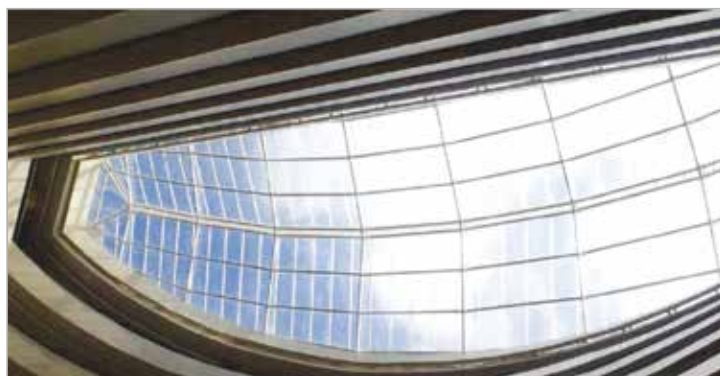
Figure 1b: Polycarbonate Sheet Roof System
