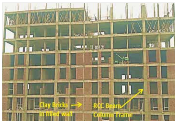
Conventional construction technology – beam column frame with brick infill wall
