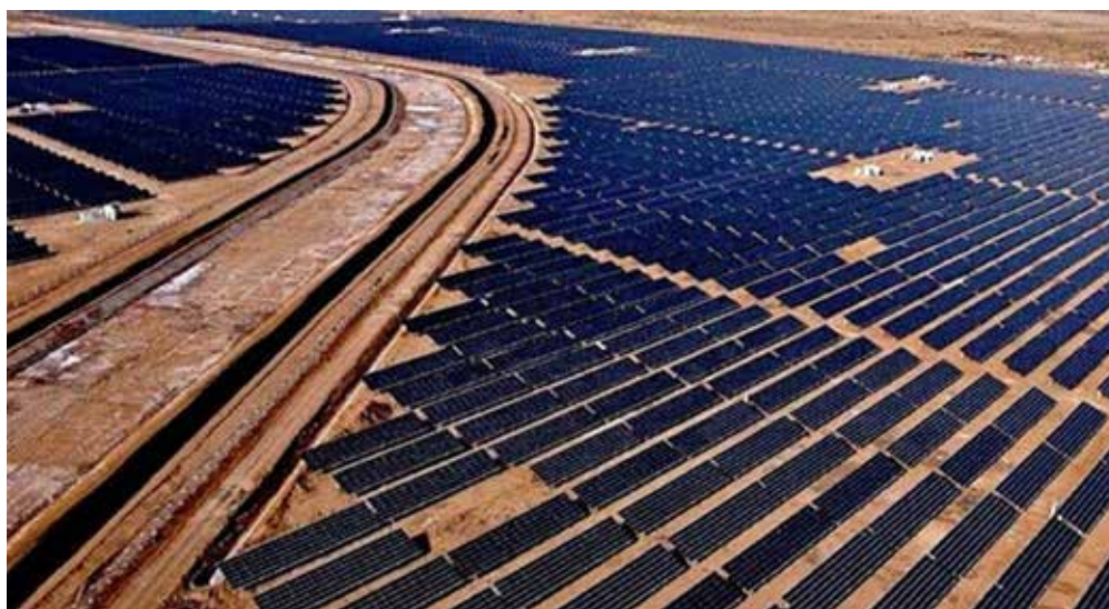
Adani Solar Plant at Kamuthi, Tamilnadu
