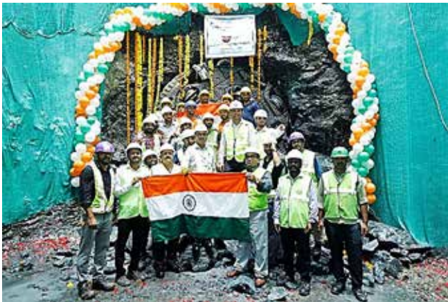
Photo-2: Breakthrough of 4.6 km tunnel crossing Tungareshwar Wildlife Sanctuary
