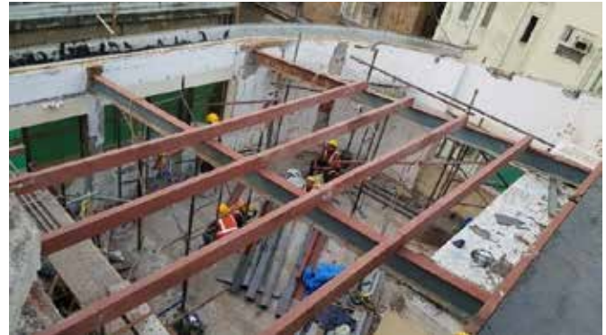
Figure-1: Strengthening the Floor System
