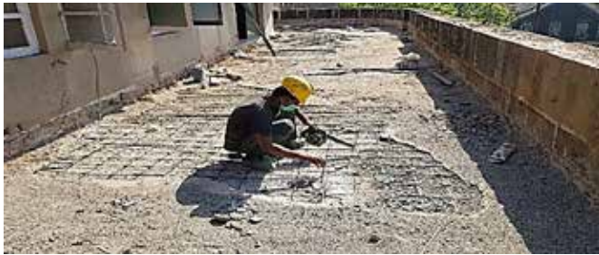
Figure-5: Repairing a Roof
