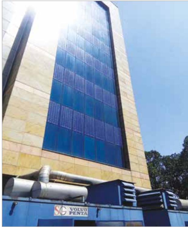
Figure-7: TCE Office building, Jamshedpur: BIPV panels
