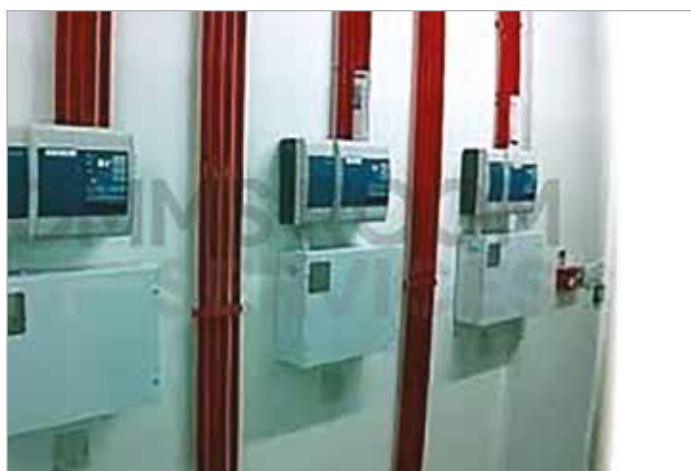
Smoke Aspiration System - Addressable intelligent spot type laser detector with sensitivity 50 times higher than photoelectric detectors
