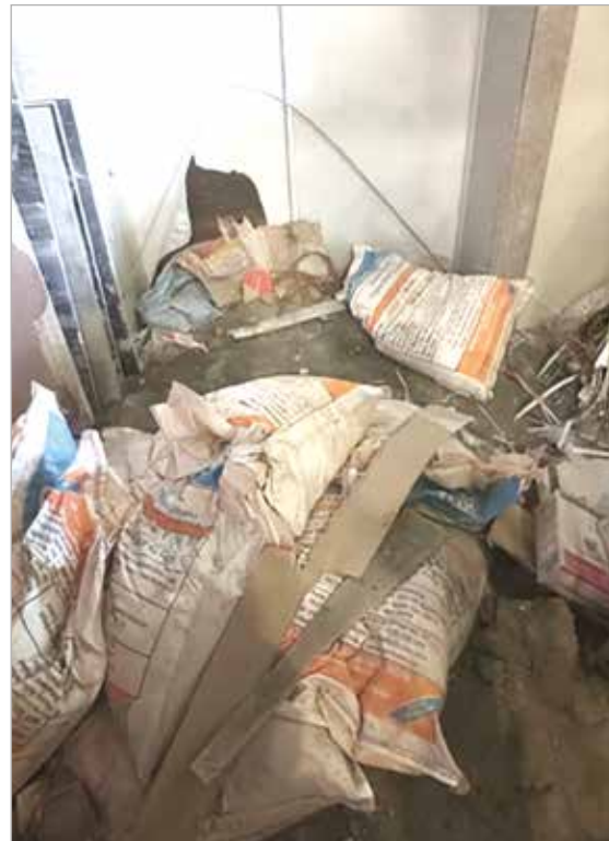
Elevator lobby with debris stacked against the door
