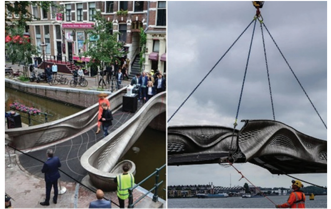
Figure- 4: 3D-Printing technology in Bridge Engineering
