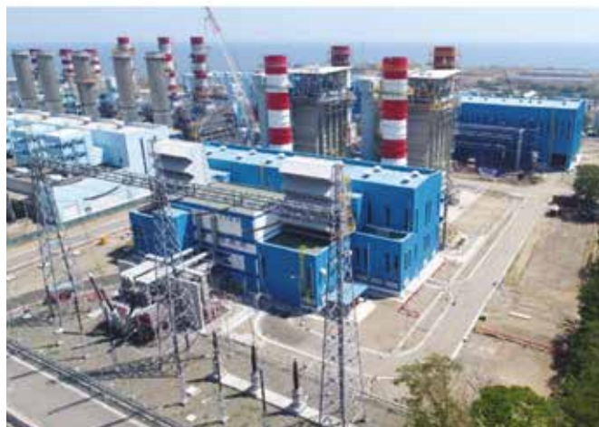
Figure-1: Bird's Eye-view of Completed Plant
