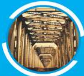
Bridges, Flyovers, Interchanges and Other Structures
